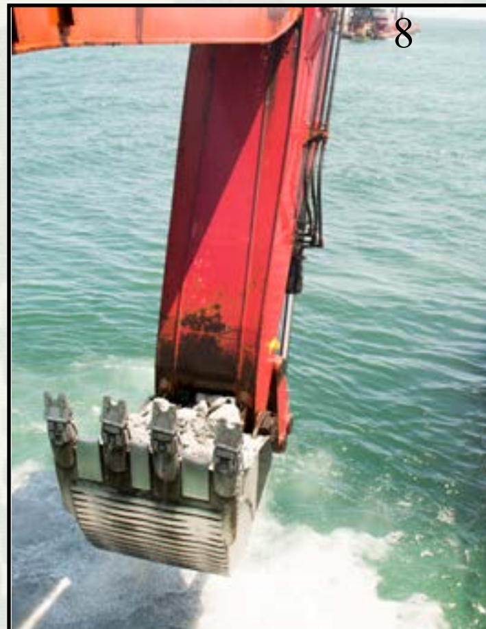
On the cover: The Charleston District is constructing reefs with the hard bottom material dredged from the Charleston Harbor's Entrance Channel. The bucket drops hard bottom material onto the scow, which transports the material to the reef construction sites.
