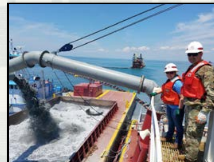
Lt. Col. Jeff Palazzini stands with Holly Carpenter, Post 45 project manager, looking over the scow where dredged material from the Entrance Channel is pumped.
